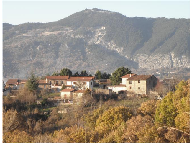
Figure 9. Building roof orientation to the south offers the possibility to use it for the installation of photovoltaic panels.
