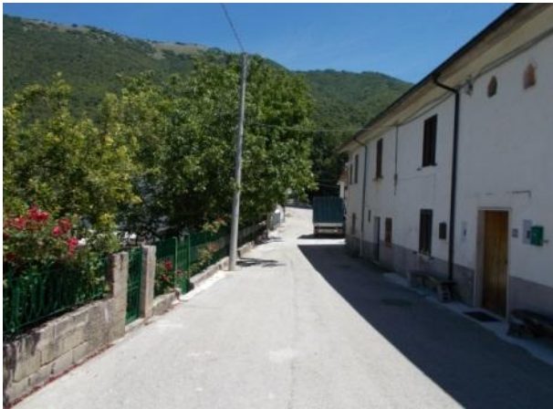
Figure 4. Typical terraced houses built in Alzano after the earthquake of 1915.
